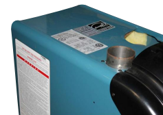
ESC boiler rating label location
