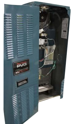
PVG/SCG boiler rating label location.
